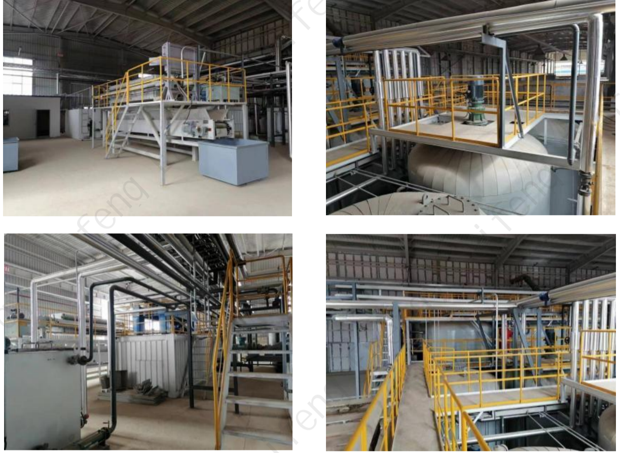
Case 4: Oil Sludge Reduction Project in Daqing
