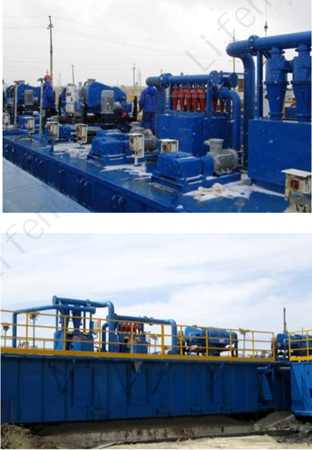
Case 3: Oil Sludge Reduction Project in Daqing
